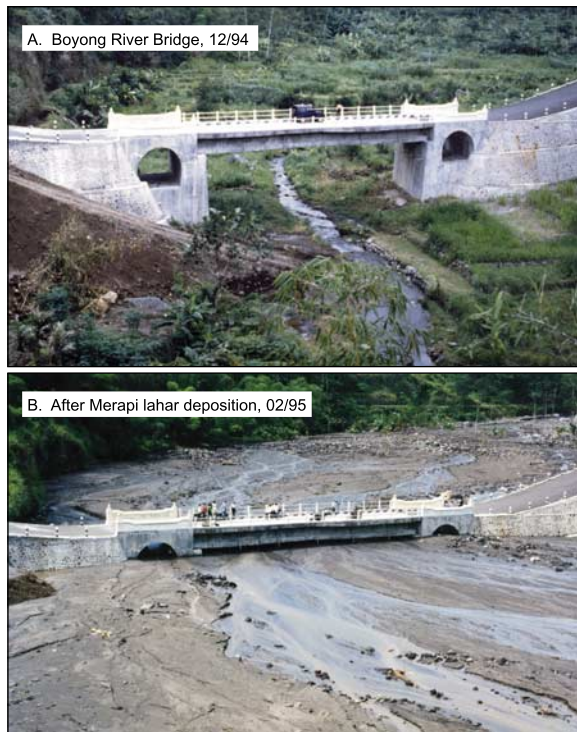
Figure 2. Example of a lahar deposition zone on the south flank of Merapi volcano, photographed at the Boyong River Bridge at three months time distance (courtesy of F. Lavigne). (a) Land-used flanks of the valley in December 1994. (b) Volcaniclastic sediment deposition photographed in February 1995. This example illustrates the fast sedimentation rates and deposition of unconsolidated volcaniclastic material, the sites of which may be especially dangerous during an earthquake. For more details about this site see Lavigne et al. [2000].
